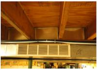
Duct leakage is a major energy-waster in buildings where the ducts reside outside the home’s thermal boundary in a crawl space, attic, attached garage, or unconditioned basement. When these intermediate zones remain outside the thermal boundary after weatherization, duct sealing is usually cost-effective.
